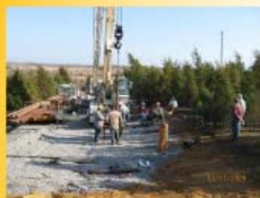
Greenville well during preparation for aquifer test.
